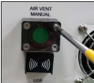
Figure 14 Remove Phillips screws
